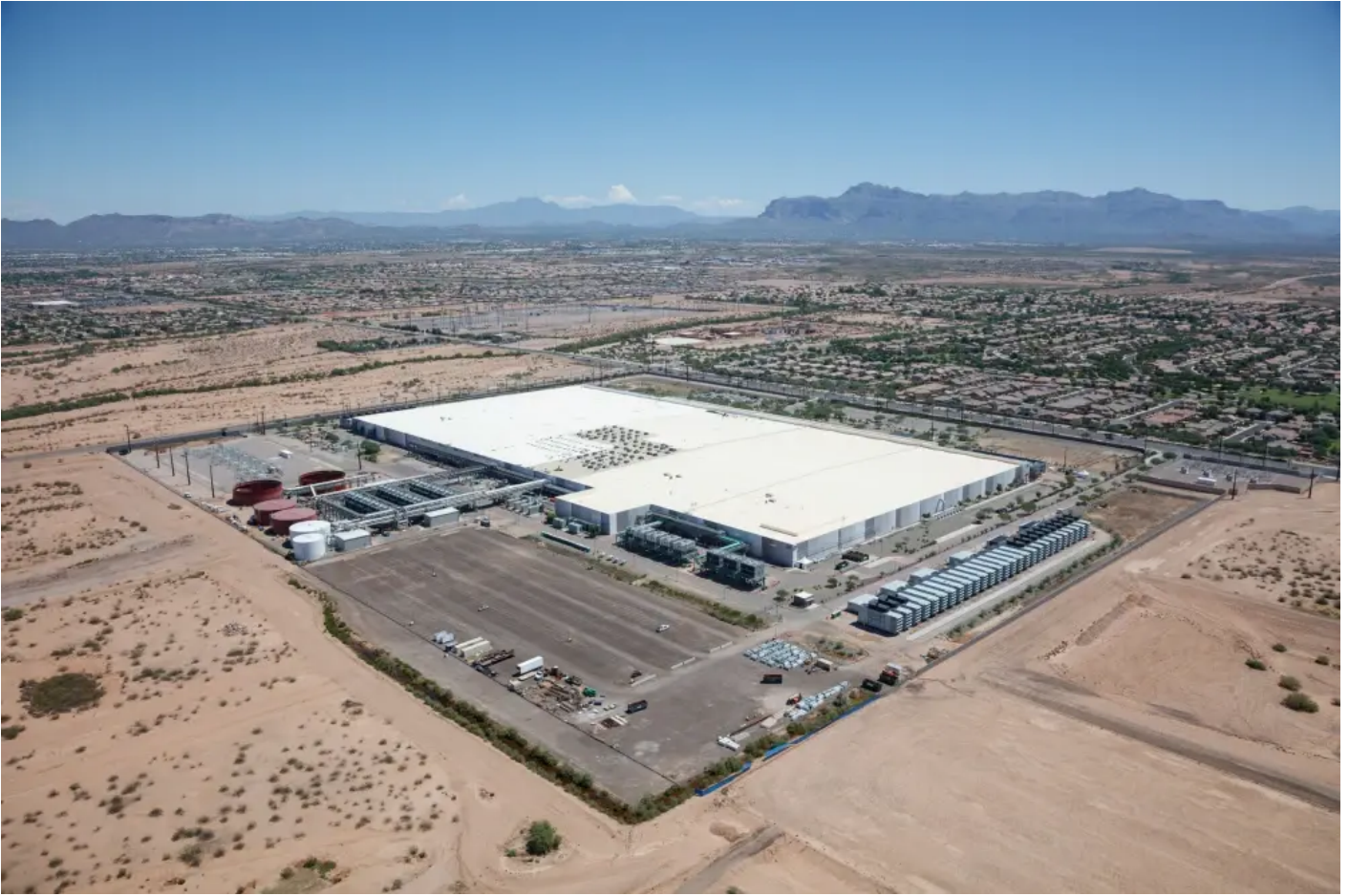
Image: Apple's data center in Mesa, Arizona
