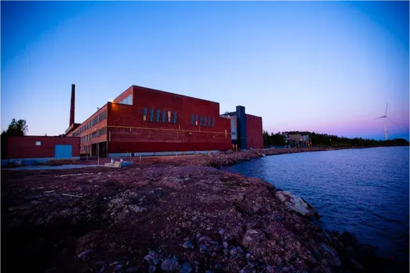
Image: A Google data center in Finland that utilizes seawater cooling
