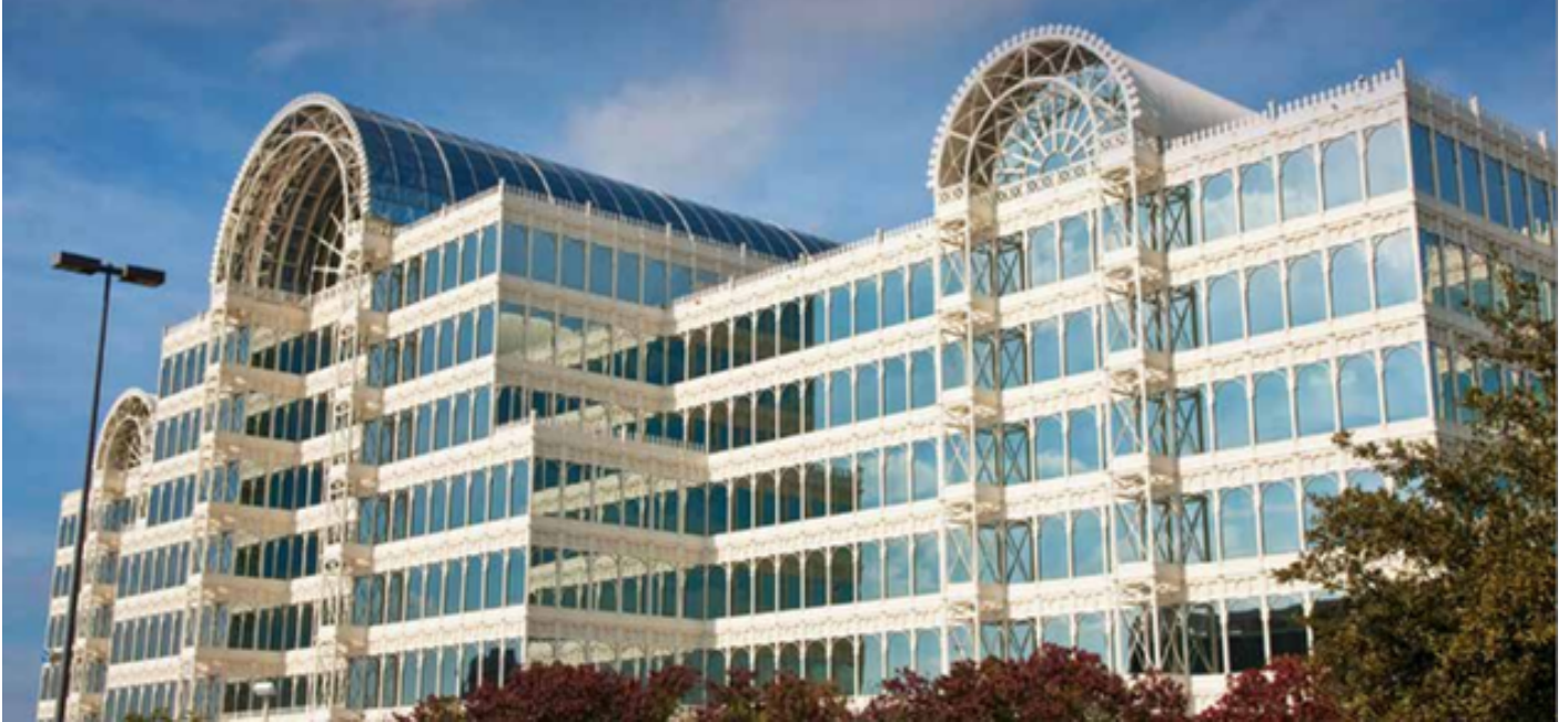
Equinix Data Center in Dallas, Texas
